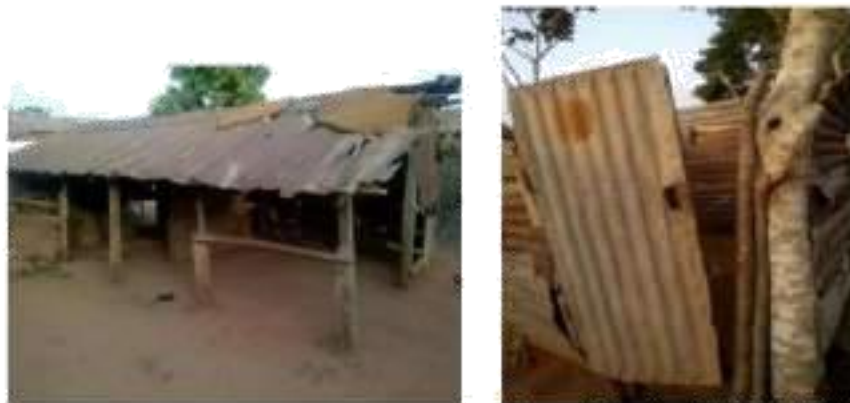
Plate 5: A set of make-shift Kitchen and Bathroom within the study area
