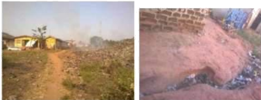
a b Plate. 4: Heap of Refuse at the Igbo Ewe site (central portion of study area) in 'a', while 'b' depicts typical erosion course converted to refuse dump in Ona Osi Quarters
